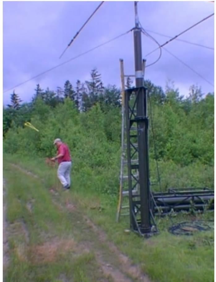
Fran (KM1Z) walking the 40 meter full wave delta loop antenna out away from the AB-577/GRC military surplus crankup tower with Fran's A3S tribander on board
